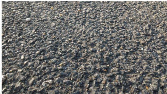
Old asphalt concrete with worn out bitumen
